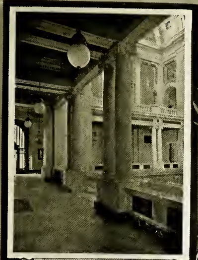
SECOND FLOOR GALLERY
